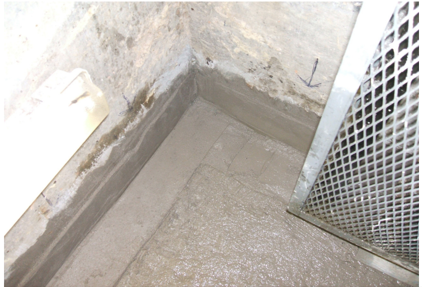
A finished lift pit using injection waterproofing
