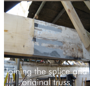
Timber Resin Splice
