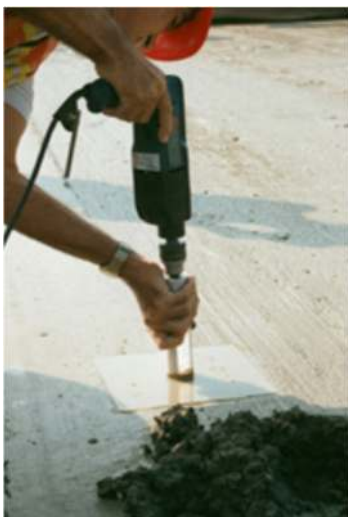
Taking a concrete
